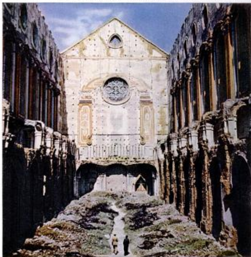
STA. CHIARA CHURCH IN NAPLES, built in 14th Century, burned after bombing and roof caved in. Decorations added in 18th Century, traces of which are visible, peeled away, revealing 14th Century rose window.
