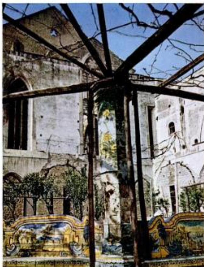
NUNS' CLOISTER of Sta. Chiara Church in Naples is braced by structure of wooden beams. All the arches in arcade were bricked up by AMG to keep building from collapsing.
